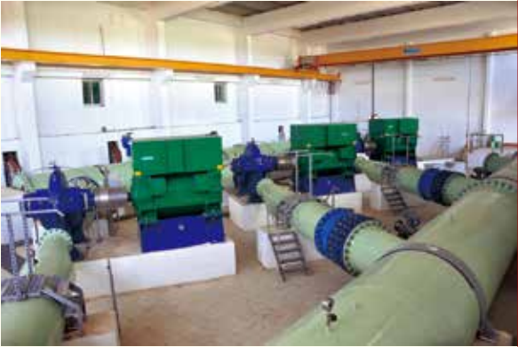
Beni Nadji 泵站设备(日输水量 150000 立方米) Beni Nadji pumping station (Capacity of 150,000 m 3 /d)
