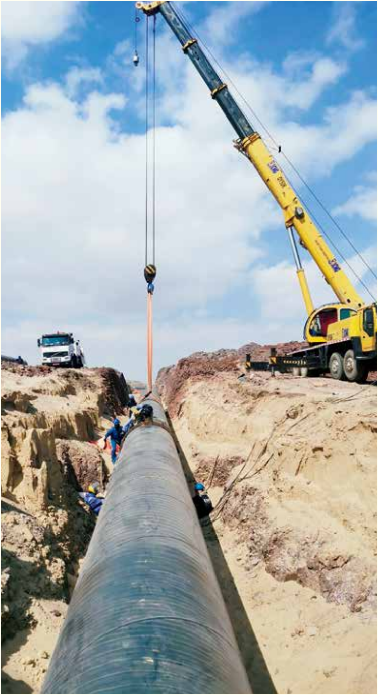
管道铺设 Laying of pipeline
