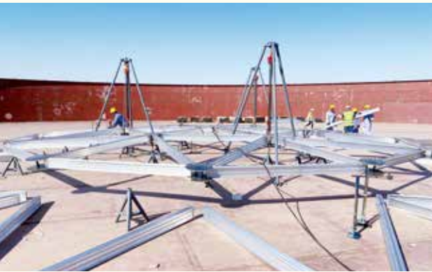
钢水池穹顶施工 Dome construction of steel tank
