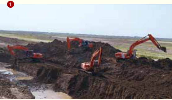
① 曝气池土方开挖 Aeration tank excavation
